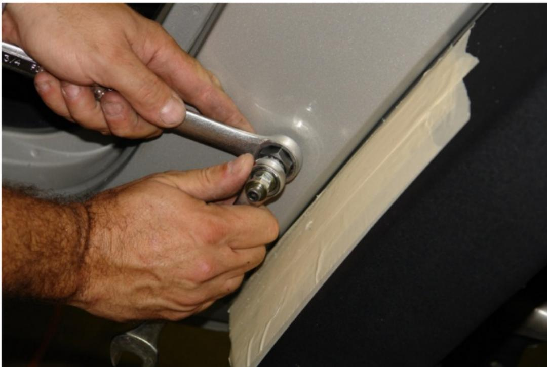
4. By turning the outer hex head, the center bolt will pull the rivet nut into a flange on the backside of the panel. In most cases, this process will have to be done twice. Continue to turn the head until the tool no longer pulls, reset the tool, and continue turning to completely seat the rivet nut.
